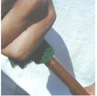
Place body over the ground rod and insert wire into metal barrel
