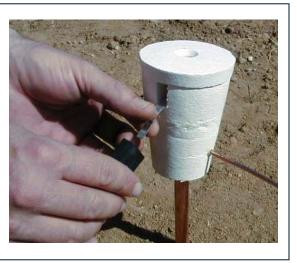
**4** Move a safe distance away from the ground rod location . Press and hold the OPERATE button until you see smoke coming out the top of the One-Sot. Let go of the button.
