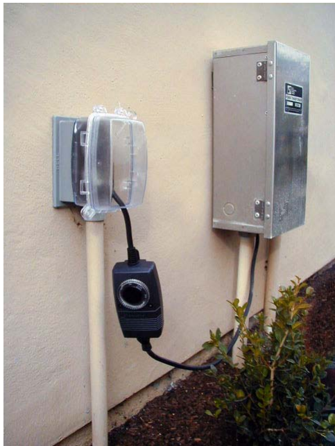
Typical NEC ® -Compliant Low Voltage Lighting Transformer installation
